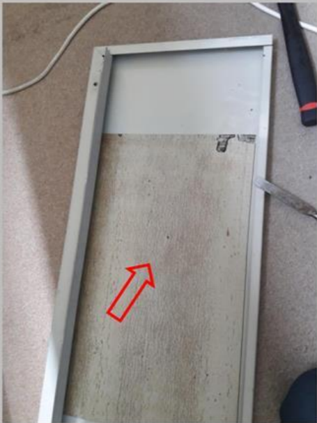
A19:radiateur- Plaque anti vibration bitumineuse
